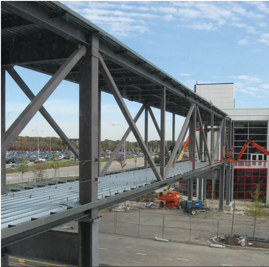
Caption: Architecturally exposed HSS sections form the verticals and diagonals of the trusses on this bridge linking the Health Careers and Natural Sciences building to the student union at the College of DuPage.
